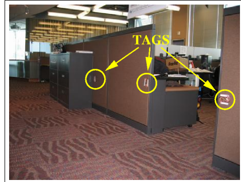
Fig. 7. RFID tags attached to walls.
